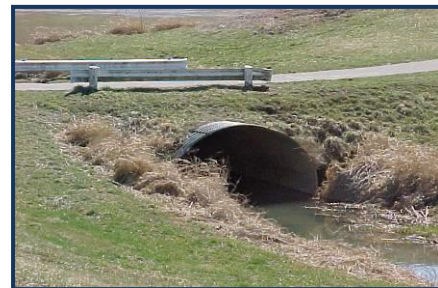
Before Mitigation and After Mitigation
