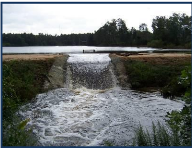
This dam failure caused flooding that damaged several homes and vehicles.
