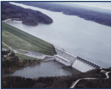
Dams vary in size and shape, the amount of water they impound, and their assigned hazard classification.
