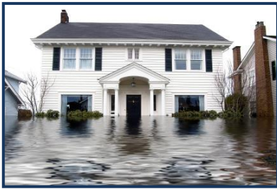
Clusters of past flood insurance claims can show where there is a repetitive flood problem.
