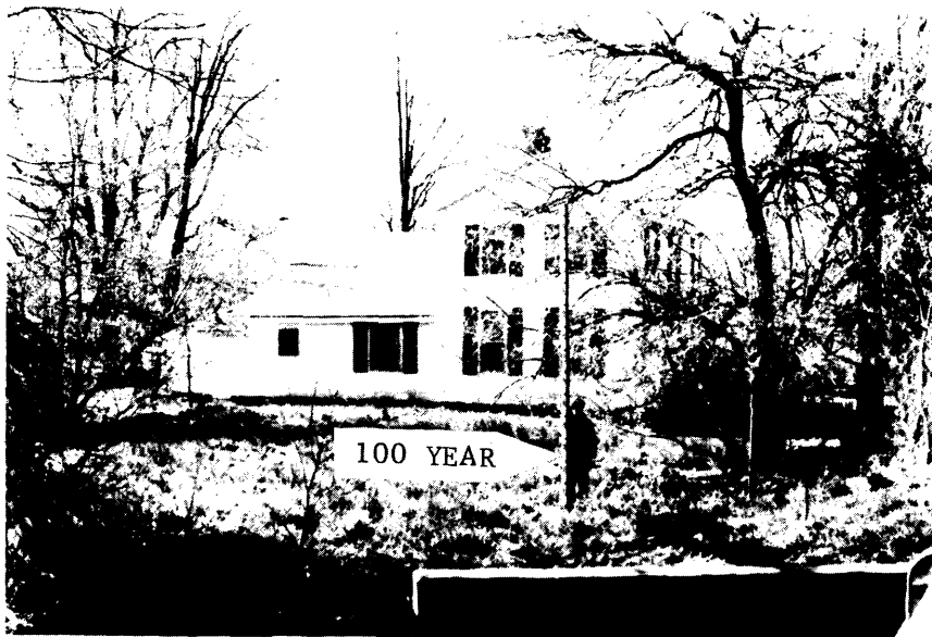
Figure 3 - At River Road bridge, Town of Leicester, projected 100-year flood elevation on Beards Creek.
