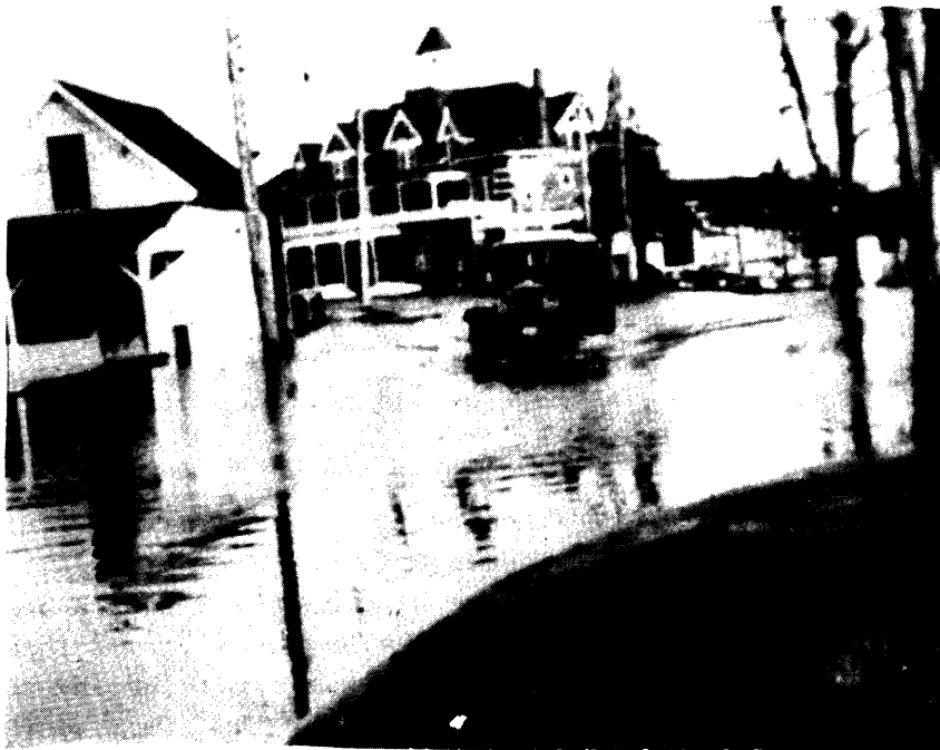
Figure 3 - Long Lake-Bay of Naples, damage in causeway area of Naples resulting from the flood of March 1936.
